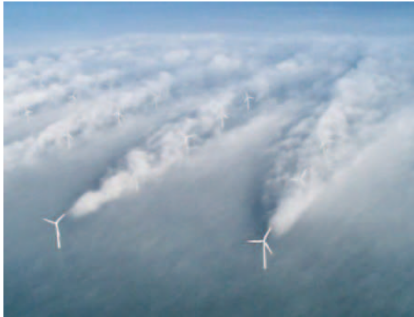
Figure 23 – Offshore wind farm. The turbulence created by the first layer of turbines is visible thanks to the condensation.
